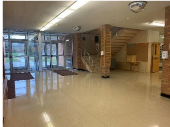
Corridor at "T" of Education Building
