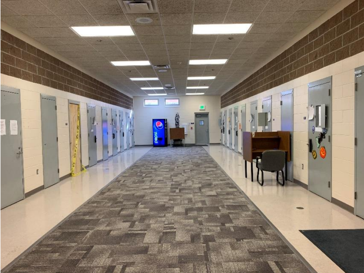
Figure 0.46 YCC | Pine Cottage Community/Dayroom with Minimal Windows
