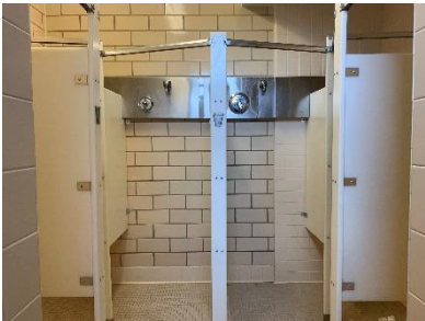
Toilet and Shower Room
