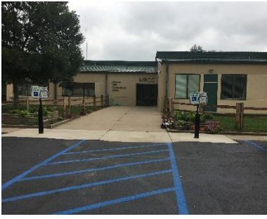
West Side-Main Building
